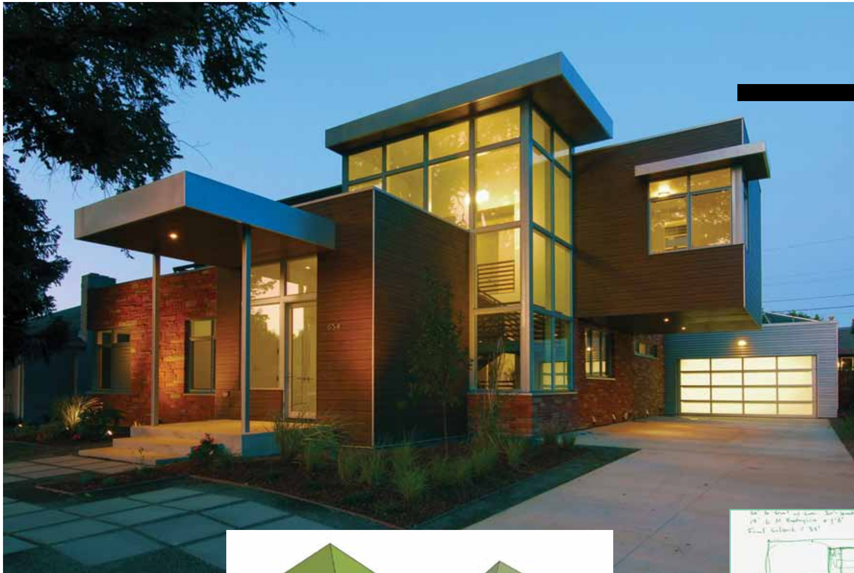
ABOVE: An exterior view of one of Elemental Living's residences on Ivanhoe Street in Denver. The stone on the exterior was reclaimed from a building on the University of Colorado's Boulder campus.
